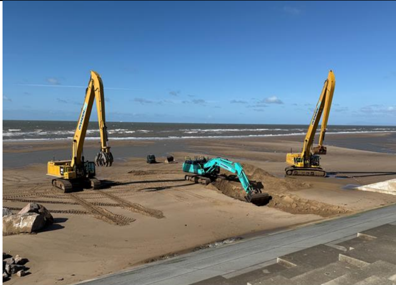
Works to prepare the beach for addition of rock armour
