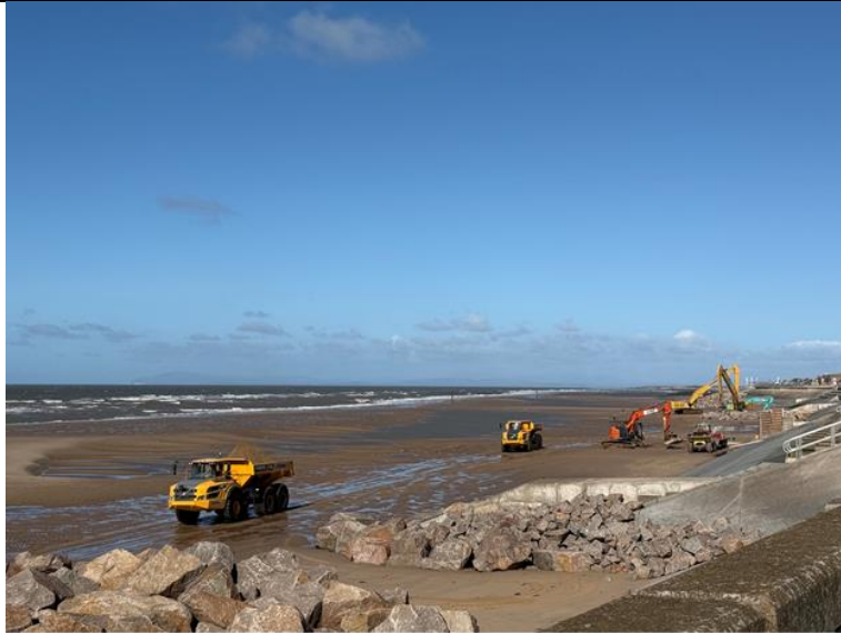
Sand being moved and rock delivered
